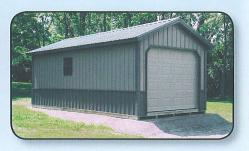
If your spot isn't perfectly level (which is often the case) we recommend that you have a rock pad installed. The rock will keep the building off the ground and if it is leveled out properly (with a laser level or by a professional) the building will sit level too.
