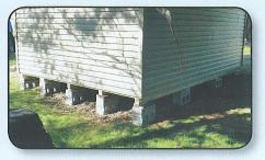
We also offer a service called Pro-blocking. It will basically do the same thing as the rock pad, but will cost less and be less hassle for you as a customer. We will place blocks under every runner and also in the middle of your building if it is longer than 8 feet. We supply the blocks.
