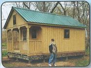
The Alpine Hideout has a steeper roof than the cabin, which makes it the right building for a loft (but with only 6'5" sidewalls). A great building for a playhouse.
