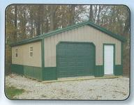
Our Clear Span Garage comes in 2 sections too, but has no walls in the middle. It has only 1 garage door, which can be put anywhere in the front gable. 8" overhangs and 1 prehung entry door are standard.
